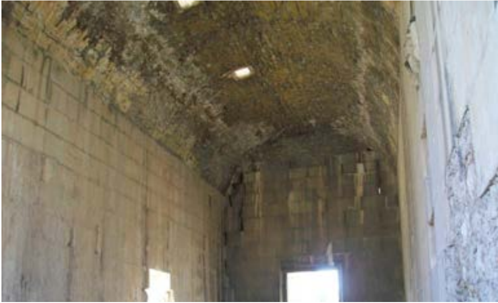
Fig. 1. Athens, Hephaisteion. Interior showing barrel vault (photo from internet)
